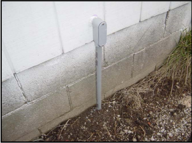
Photo© courtesy of Home Wiring USA www.selfhelpandmore.com
